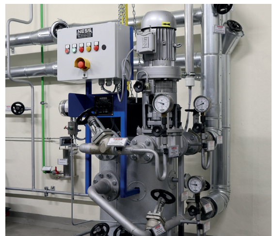
Installed Fine filter station FF300
