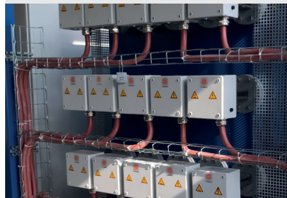
Heating flanges of EWE with 50 kW each
