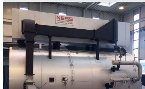
Heater with installed combustion air pre-heater (Luvo)
