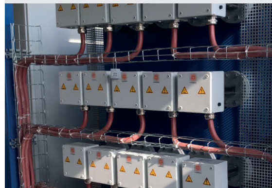
Heating flanges of EWE with 50 kW each
