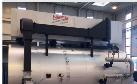
Heater with installed combustion air preheater (Luvo)
