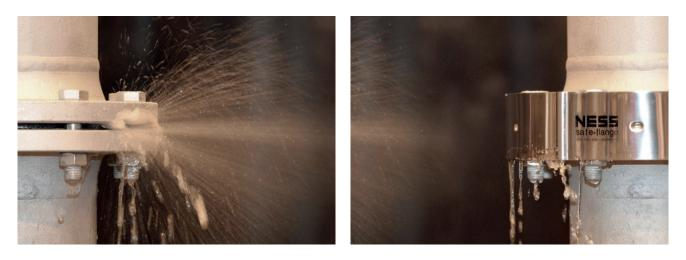
Securing pipe systems with flammable, hot, toxic or corrosive liquids and vapor is a must, especially when they are under pressure. If leaks occur on the flange connections, liquids can splash through the room and severely endanger employees and systems.
