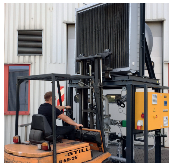
Two-part skid designed for forklift transport
