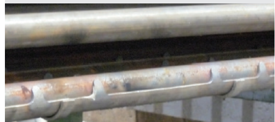
NESS Protective shells are fixed on the pipes to be protected
