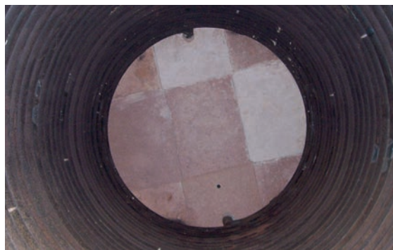
Heater back wall shown with lightweight refractory concrete
